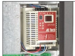
variable speed motor drive
